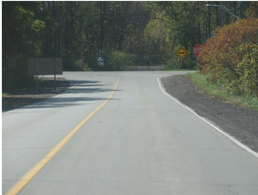
FIGURE 6: Reid Side Road Approach to Twiss Road
